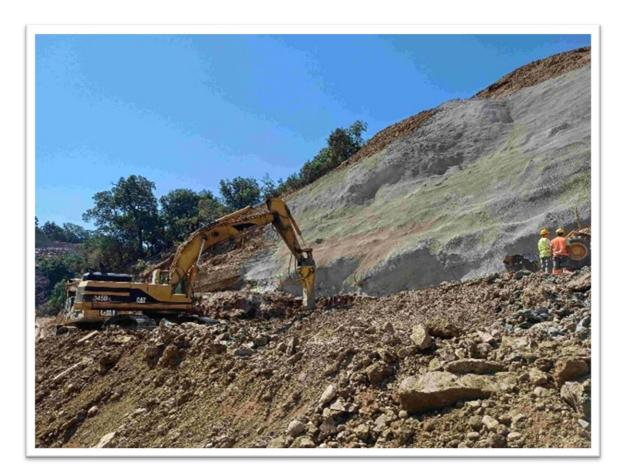
Removal works of loose materials, lean concrete, anchors & shotcrete at the Right Buttress, 7/2025
