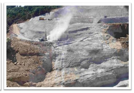
Excavation and removal works of loose materials of the bedrock on Dam's base, 10/2025
