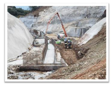
Installation of steel reinforcement for stream's diversion & Outlet - Ecological Flow Conduit
