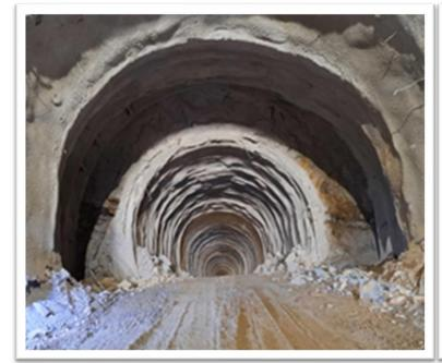
**Excavation works and implementation of the temporary support measures**
